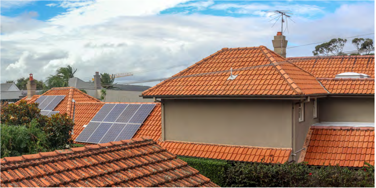
Viewpoint no.35: Existing site photo. From balcony off main living room at No. 45, Muston Street, looking E/N/E towards subject site. From a standing position.
